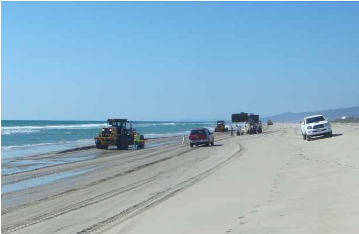
**Figure 2:** The beach route was prepared using graders and bulldozers below the mean high tide line to create an even driving surface for the crawler.
