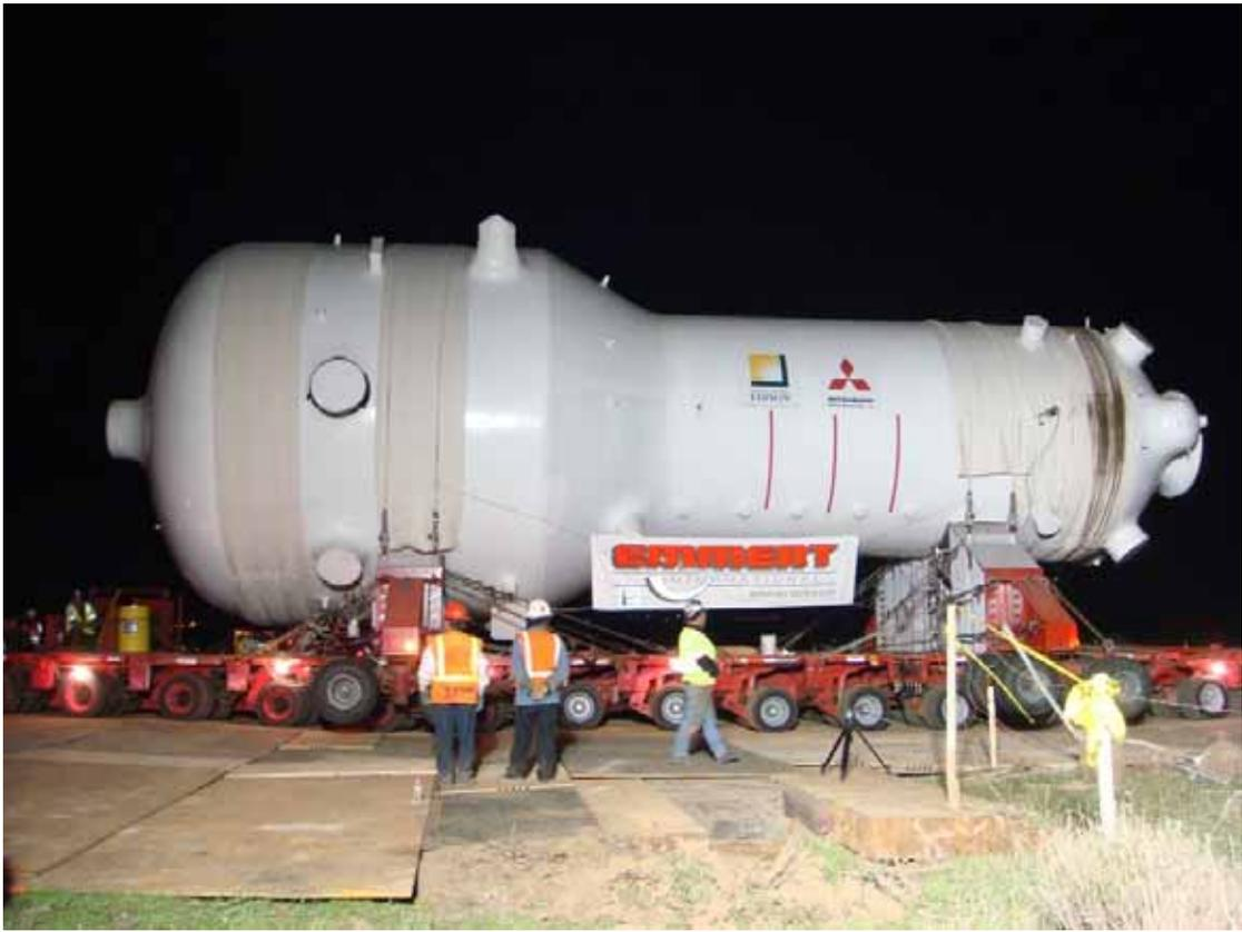
**Figure 5:** RSG transport along Interstate 5 on the Goldhofer. Steel plates were used to protect curbs and pavement.
