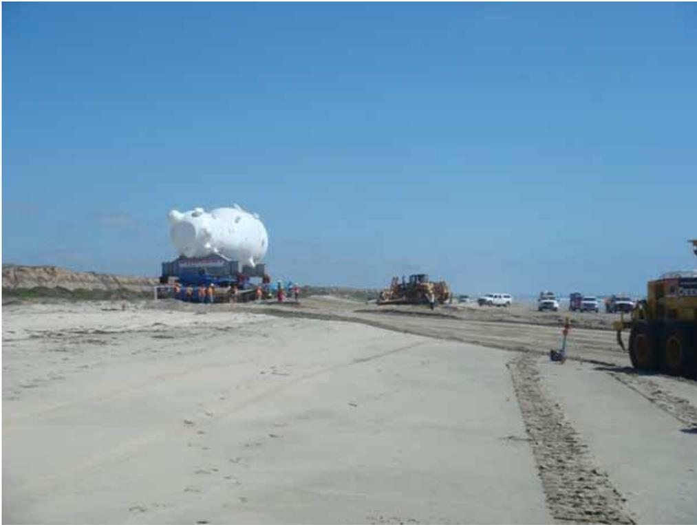
**Figure 3:** The RSG at a layover area above the mean high tide line along the beach route. The RSG was staged overnight in the layover areas and resumed transport during the next low tide. Ramps created for RSG access/egress were re-contoured after use.
